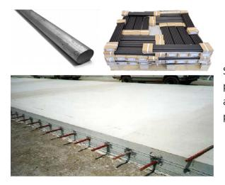
Smooth dowels are placed in concrete slabs to enable proper load transfer across the joint, maintain vertical alignment of the slabs, and allow slab movements perpendicular to the joint.
